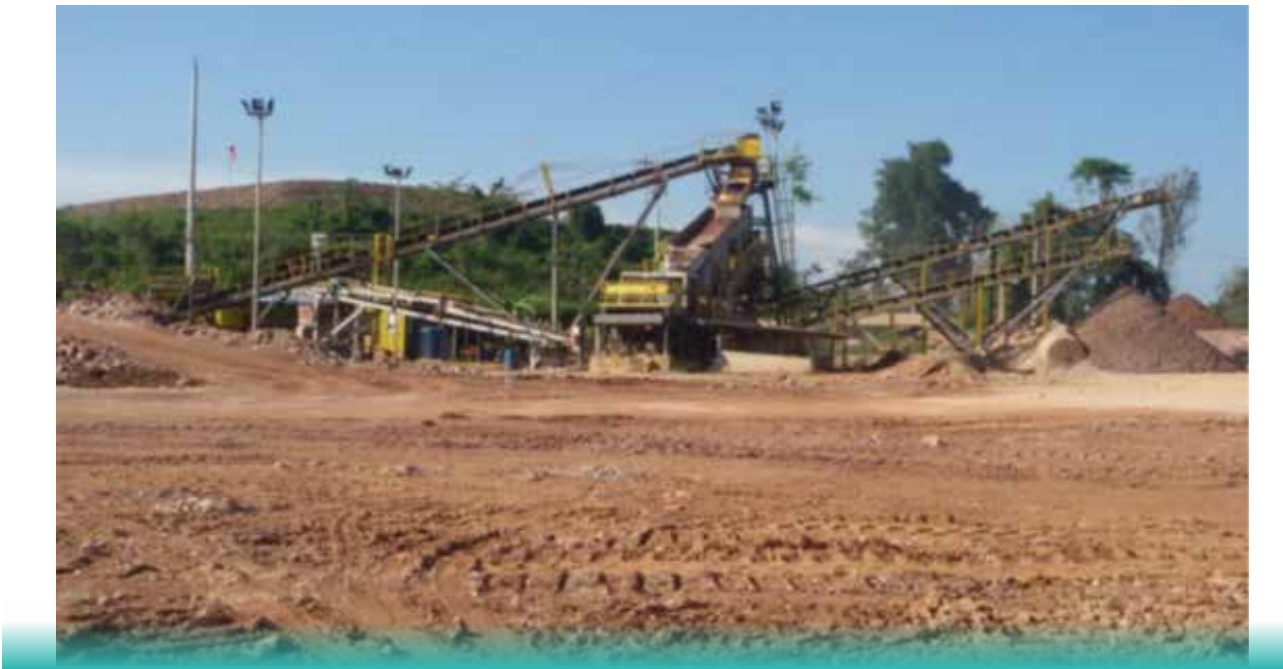
Proses Crushing Bijih di Perseroan | Ore Crushing Process in the Company
